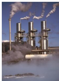
Svartsengi geothermal power plant, Iceland.
