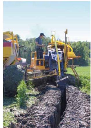
▲ When a lime filter ditch is installed, the lime is mixed into the backfilled soil. The lime binds phosphorus that is dissolved in the water.
