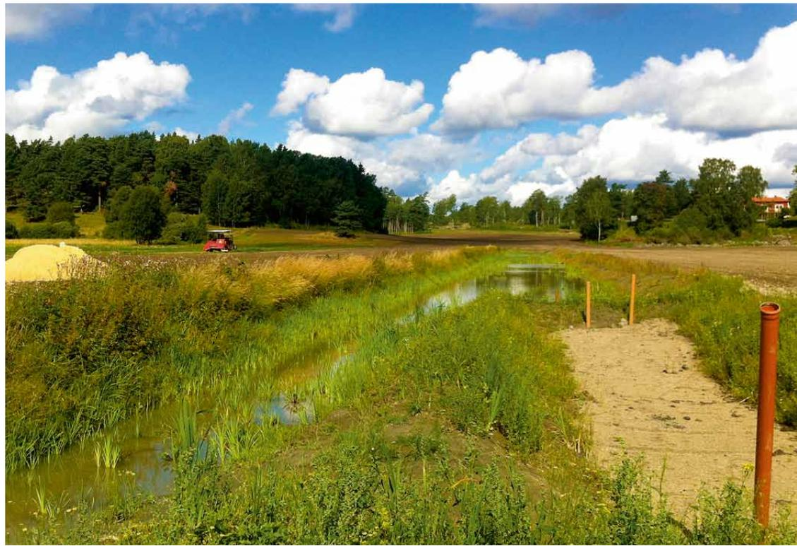
▲ At Säby Farm at Björnöfjärden, structure liming and phosphorus ponds with lime-filter beds, among other measures, have reduced the nutrient load from agriculture to the bay by just over 80 per cent. In the middle of the picture, the narrow phosphorus pond is visible with the lime filter bed on the right. To the left of the pond is a pile of structure lime to be incorporated into the clay field.
